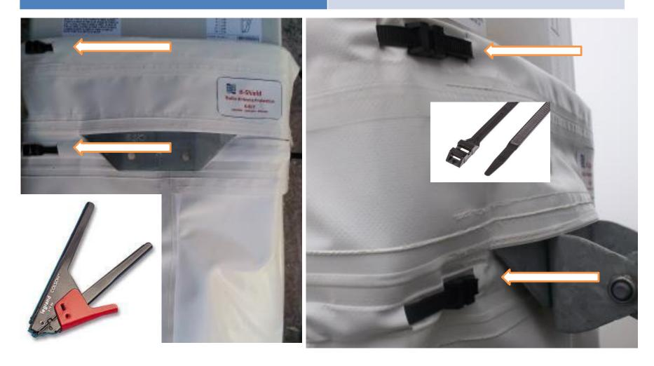
Step 6: Tie the bottom of the Antenna.
