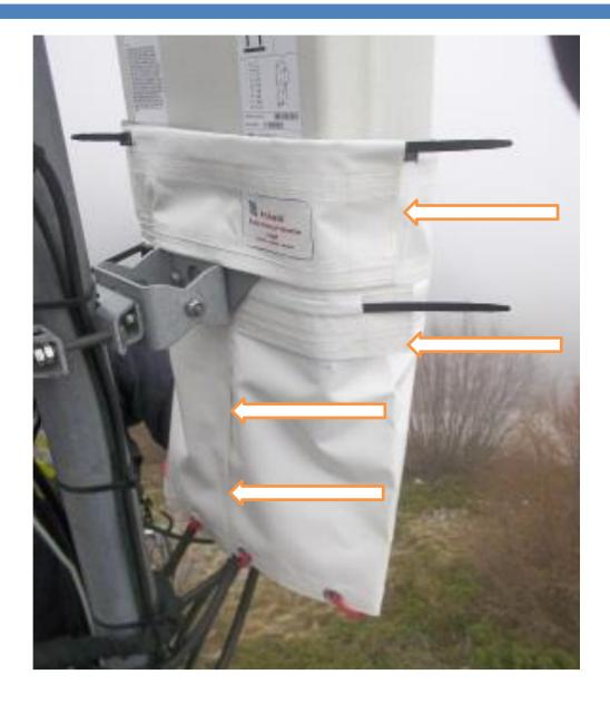
Step 5: Fasten the plastic Ties using Tie Crip Fasten tool.
