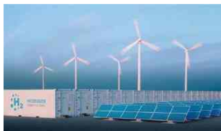
Hydrogen production station
