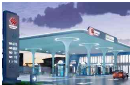
Hydrogen refueling station
